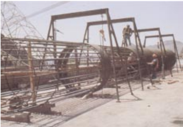
Front end of the parking structure is founded on huge concrete caissons sunk to depths of 90 ft. Here workers assemble a steel cage for one of them.
