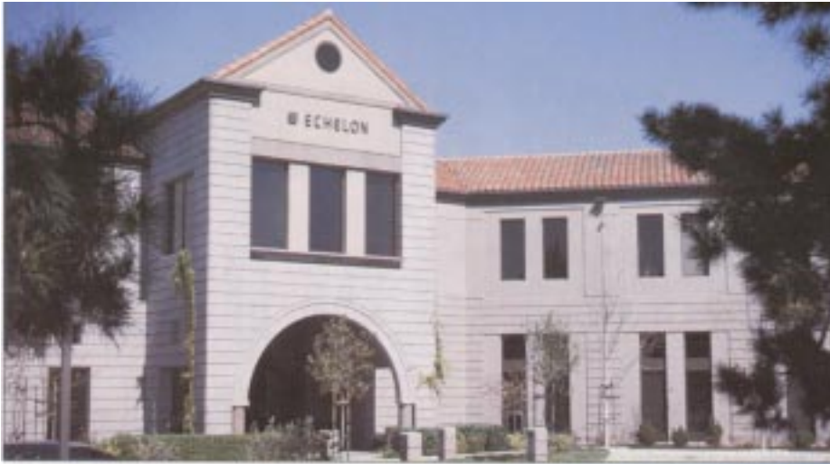
Northern California's Central Concrete applied its usual tight quality control in delivering integrally colored mixes for the Echelon Building in Pal Alto, a recent tilt-up job with general contractor Devcon. (Photo: Davis Colors)
