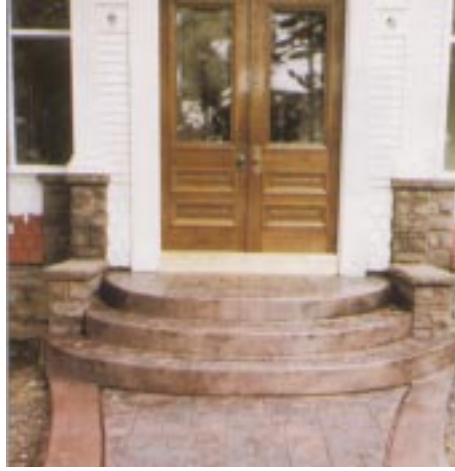
Pine Hill Concrete Mix Customer, Broad Spectrum Concrete, blends new integrally colored, patterned stamped flatwork and steps with vintage masonry.
