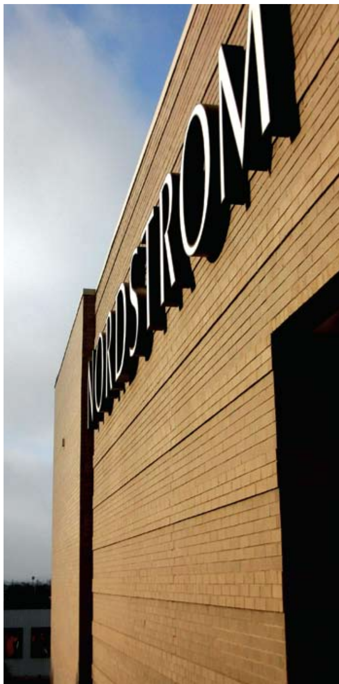
Fig. 6. With care and cooperation, consistent mortar color producing the appearance desired by the owner can be achieved.
