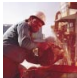
Mix-Ready bags end the dirty looks from drivers with dust in their faces, and from dispatchers upset that measuring and adding color the old-fashioned way delays trucks.
