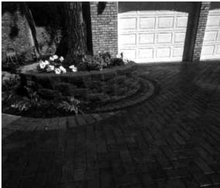
Figure 1. Many sealers enhance the appearance of concrete pavers and protect against staining.
