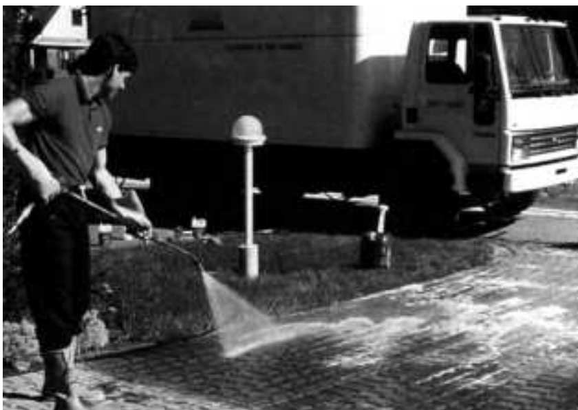
Figure 2. Pressurized cleaning equipment used by professional cleaning and sealing companies can bring out the best appearance from pavers.
