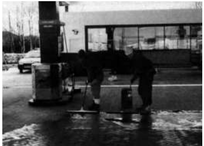
Figure 5 (above left) and Figure 6 (above right). Urethane is applied with squeegees to stabilize joint sand between pavers in aircraft pavement and at a gas station.
