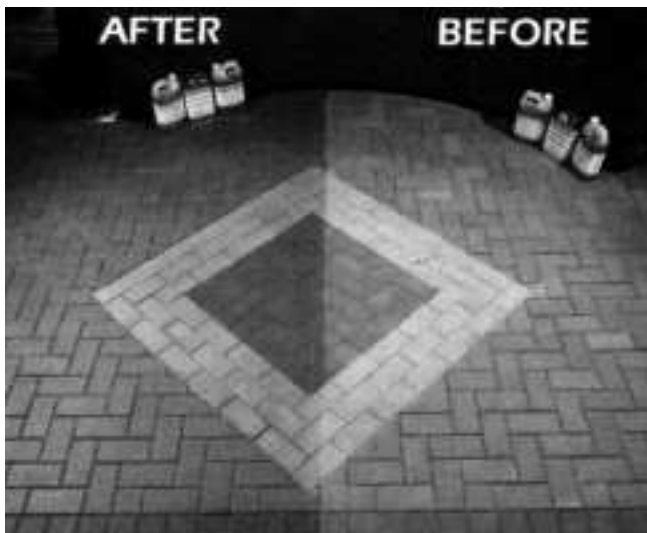
Figure 3. Before and after application of an acrylic sealer shows how it deepens the appearance of concrete pavers.
