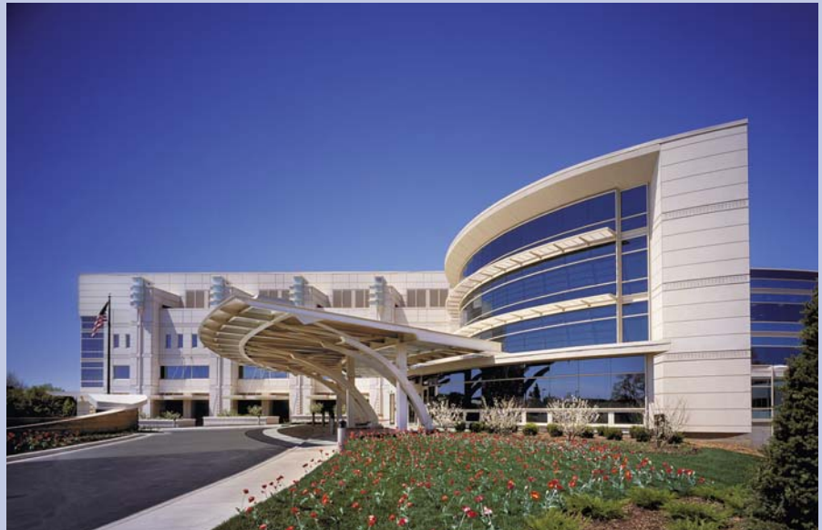
Figure 1. The Condell Medical Center is built with load-bearing precast concrete panels with an architectural finish achieved by using white cement. Courtesy of Condell Medical Center.
