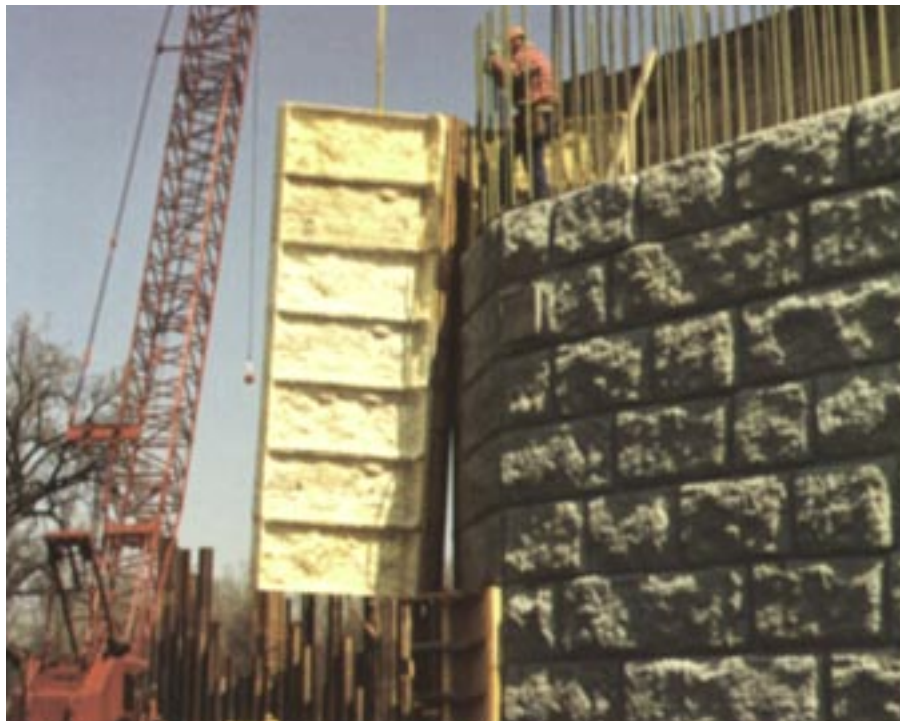
Elastomeric form liners molded from natural rock surfaces can be attached to conventional form panel and can be used to create a variety of patterns. The finished concrete surface has a realistic stone texture, with up to 10 in. (250 mm) of relief possible.
